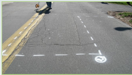
Typical survey paint markings
