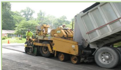
Typical hot mix asphalt paving operation
